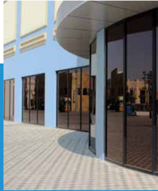
Project: River Park Client: Dubai Park & Resort Contractor: Zebian Aluminium & Glass Industry Location: UAE
