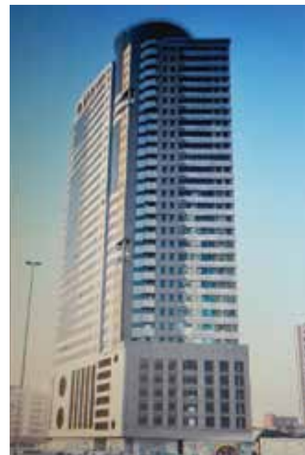
Project: Residential Building Contractor: Al Aweer Consultant: Mazaya Location: UAE
