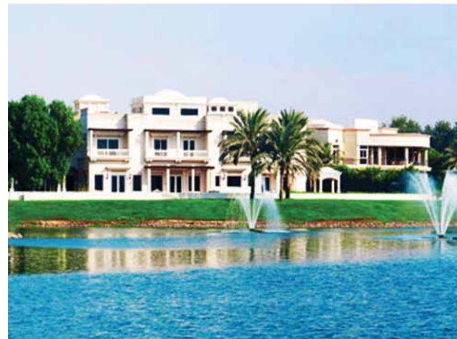
Project: Emirates Hills 76 Luxury Villas Client: Emaar Properties Consultant: Ziki Homsy Contractor: Dubai Civil Engineering Location: UAE
