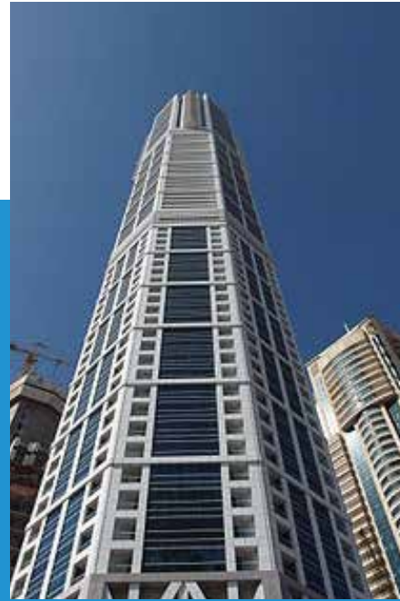
Project: Dubai Marina Tower 23 - 4B+G+90 Client: Hircon International Consultant: Keo Contractor: Dubai Civil Engineering Location: UAE
