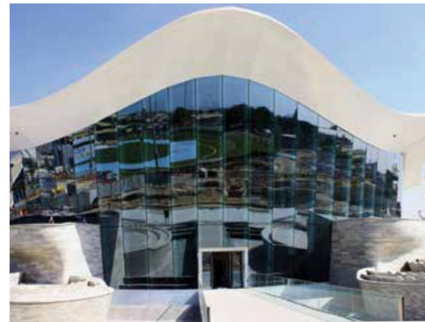
Project: PDP Contractor: Zebian Aluminium & Glass Industry Location: UAE
