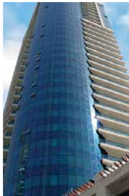
Project: Time Palace Tower Client: Abraj Frz Consultant: M3ar Architects Contractor: Dubai Civil Engineering Location: UAE
