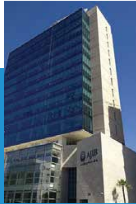
Project: AJIB Client: Arab Jordan Investment Bank PLC Consultant: Arabtech Jordaneh Contractor: Al Hamad Contracting Co. Location: JORDAN
