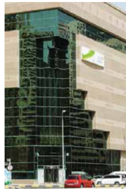
Project: Etisalat Office Client: Etislat Consultant: Al Rostamani Contractor: Al Hamad Contracting Co. Location: UAE
