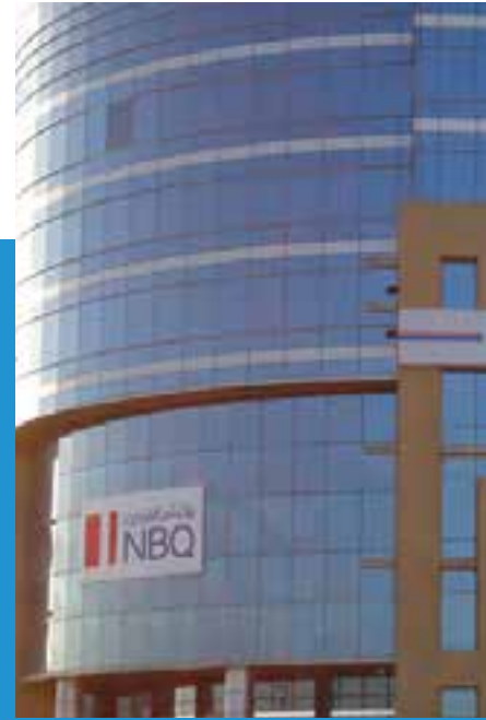
Project: Umm Al Quwain Bank Head Quarter Client: Umm Al Quwain Bank Consultant: Arenco Contractor: Al Hamad Construction & Development Location: UAE
