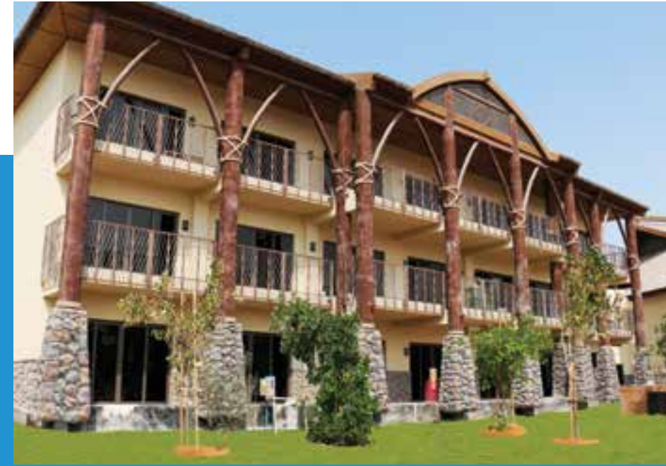
Project: Lapita Theme Park Hotel Client: Marriot Contractor: Zebian Aluminium & Glass Industry Location: UAE
